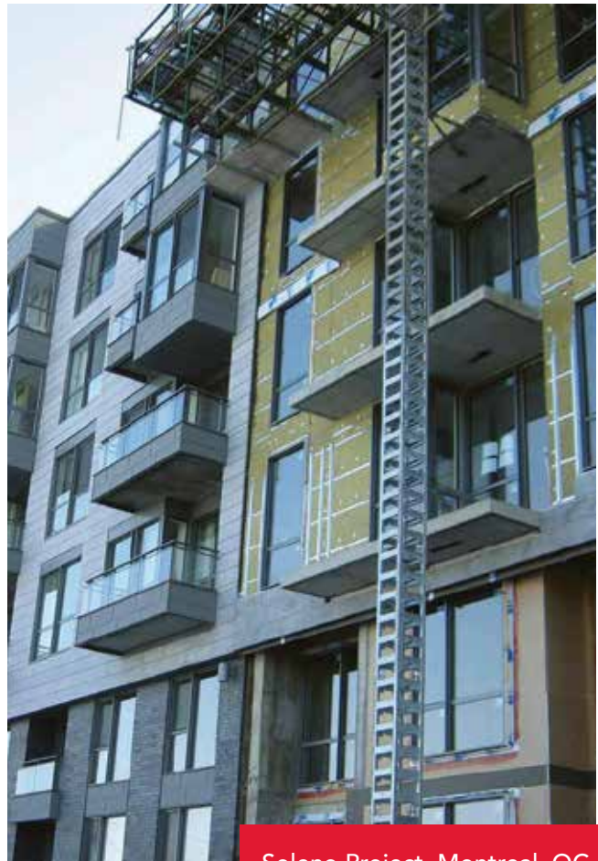
Soleno Project, Montreal, QC ROCKWOOL Cavityrock®
