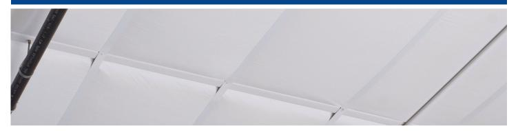
Facings for Metal Building Insulation are high quality vapor retarders. However, the facings may become damaged over the years due to accidental punctures &/or penetrations, which can compromise its intended performance. When discovered, the damaged facing must be sealed properly using a tape that has the same or better vapor retarder qualities as the facing. This ensures that the integrity of the vapor retarder facing on the insulation is maintained within the building.
