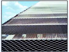
The Sky-Web II<sup>®</sup> System requires no action by workers; e.g., tying off with lanyards. Its concept is similar to automobile air bags (a passive restraint) versus seat belts (a user-operated restraint).
