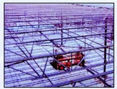
Once construction is complete, the mesh remains as a permanent part of the roof system, providing support for the insulation materials. The product's white color blends well with most fiberglass insulation facings, maintaining an attractive and nearly invisible appearance.
