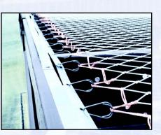
Naturally, the Sky-Web II<sup>®</sup> system cannot protect against injuries from falls onto structural members. In addition, tie-off systems are still required for workers near the perimeter of the building and during the mesh installation process.
