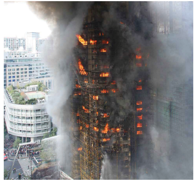
The severity of the Shanghai fire was partially a result of the use of urethane foam insulation, which aided in the spread of flame and smoke.
