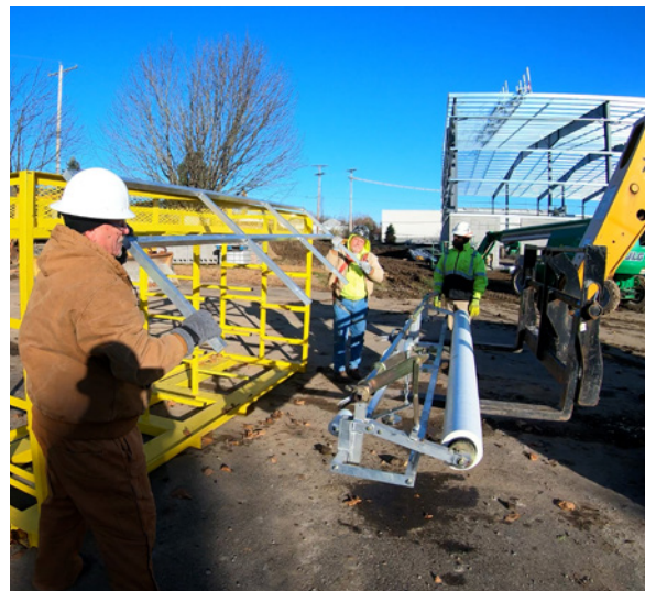
Insert the guardrails.
