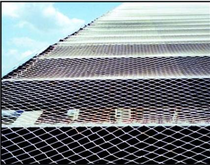
The Sky-Web II® System requires no action by workers; e.g., tying off with lanyards. Its concept is similar to automobile air bags (a passive restraint) versus seat belts (a user-operated restraint).
