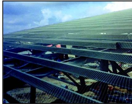
The Sky-Web II® system has a Flame Spread Index of 3 or less and a Smoke Developed Index of less than 10 as tested in accordance with U.L. 723.
